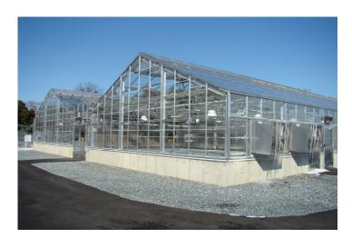
TECHNICAL SYSTEMS – High clearance interior provides stable climates. Hot water heating with all zone independents. Redundant heating system. Forced air ventilation system. Centralized cooling pad with controlled waterflow. High pressure sodium lighting system providing 200 micromoles. Shading system. Misting propagation using RO water. Bench heating system. Specialized computer control system. Fogging system.
